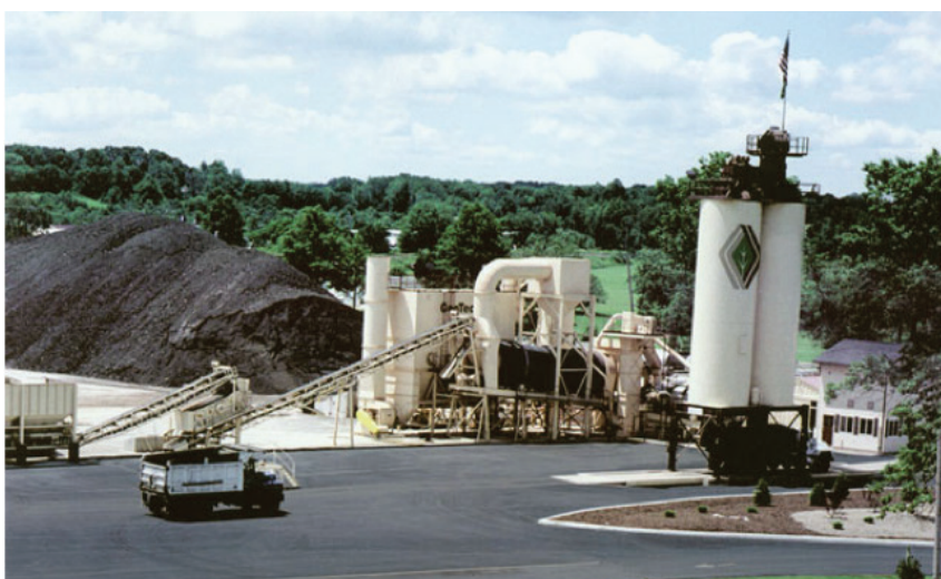
An asphalt hot plant can burn 10-20,000 gallons of LNG per day
