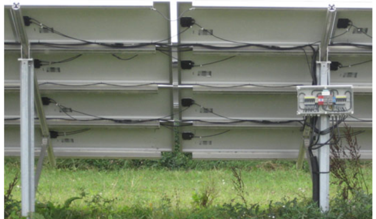
Field wiring requires costly junction boxes and is prone to failure
