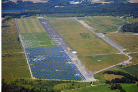
Construction status at the end of July 2007
