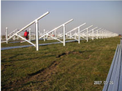
Construction of the first aluminum sub-structures for the solar modules on March 26 th , 2007
