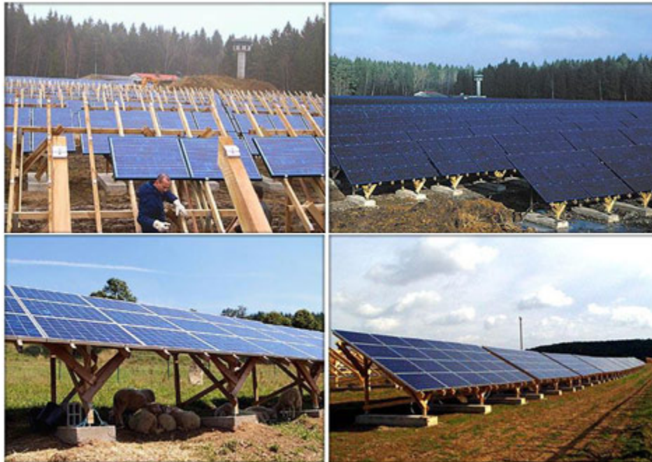
Suntechnics sites http://suntechnics.com/us/installations_2cm.htm
