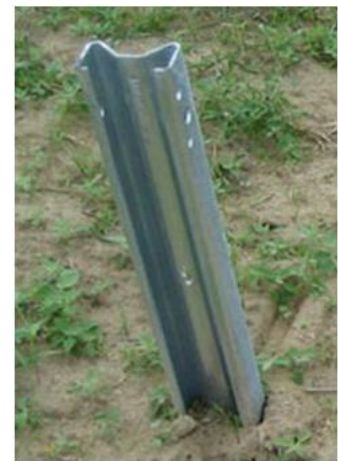
Driven post-lower unit cost
