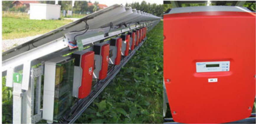
SMA string inverters at Gehrlicher Hesse site
