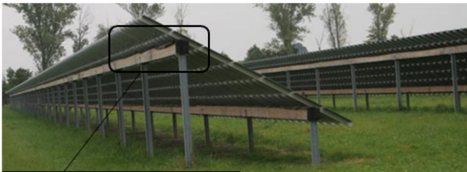
Tar paper covering laminate wood
