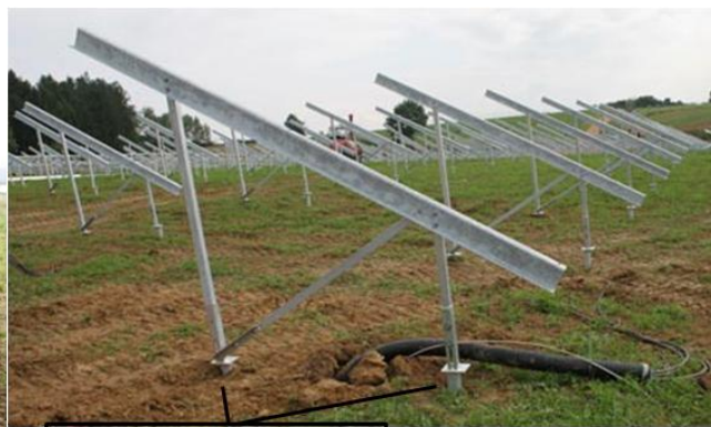
Dual earth screws - Terrafix
