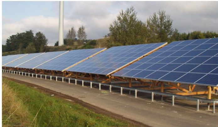
Old Wooden Racks – Juwi Solarenergie Morbach
