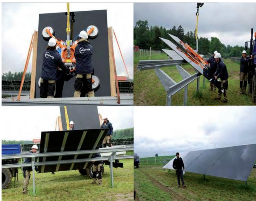
Large 5.7m 2 AMAT modules test installation by Phoenix Solar
