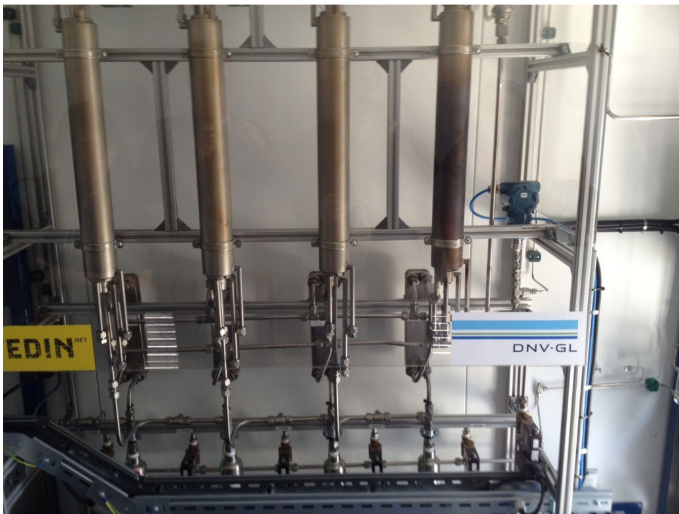
A power-to-gas facility in Rozenburg, The Netherlands. Photo credit: Jared Anderson/Breaking Energy
