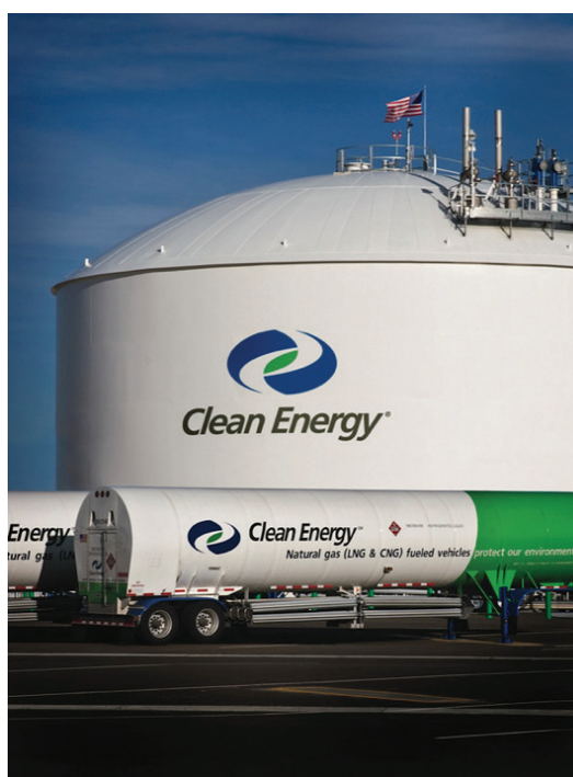
Storage and transport facility, Clean Energy Fuels Inc.
