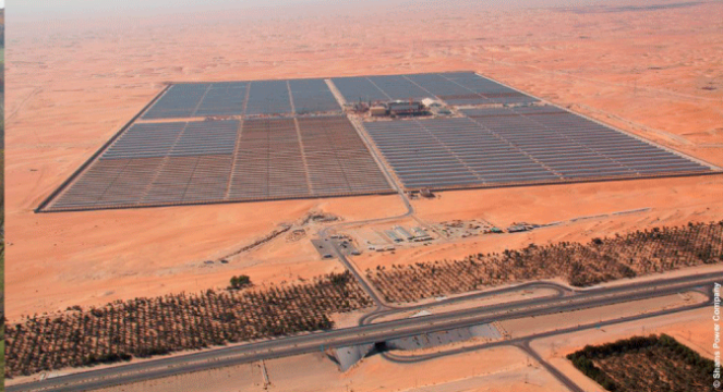
Shams 1 CSP facility in Abu Dhabi, 100 MW. Commissioned in 2013, it covers 1 square mile of desert.
