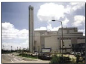
Kinuura, Japan ash vitrification facility, neutralizes ash from an MSW incinerator
