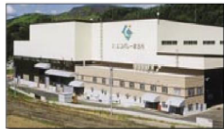
The Utashina plasma gasification facility processes up to 280 tpd of MSW & auto shredder residue and produces electricity
